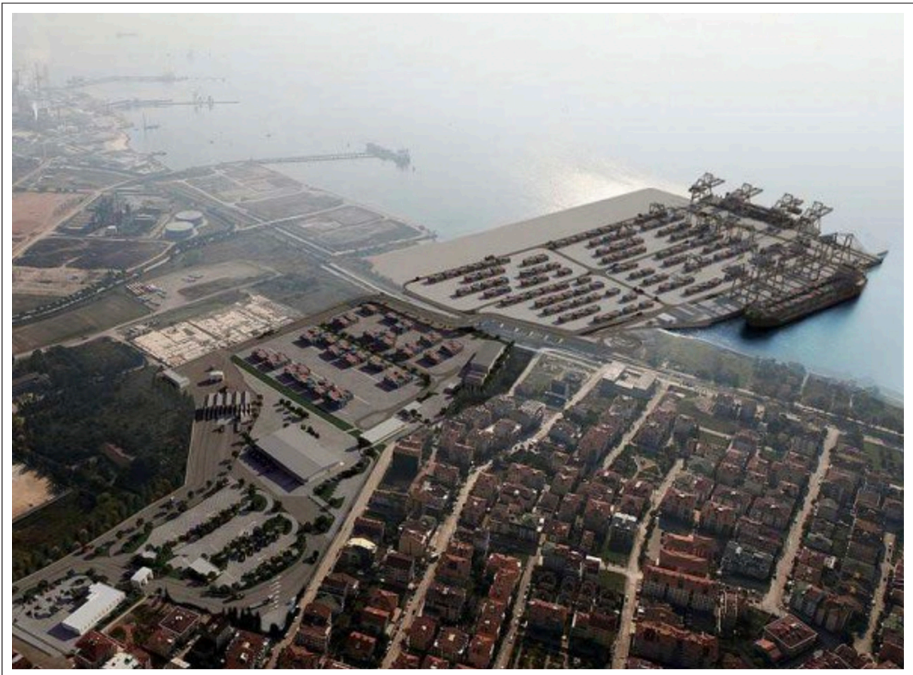
Figure 5. Completed Yarımca container terminal project.
