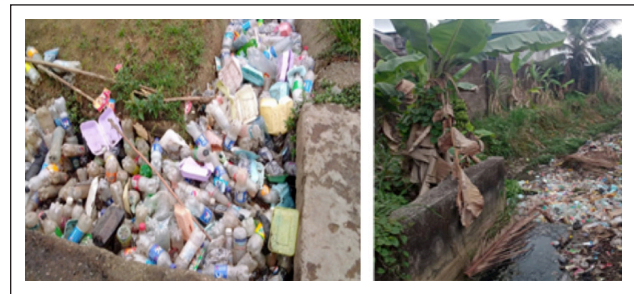
Figure 1. PET/PS blocked drains.
