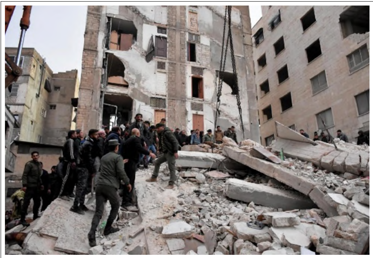
Figure 3. The collapsed 8-storey building in Hama.
