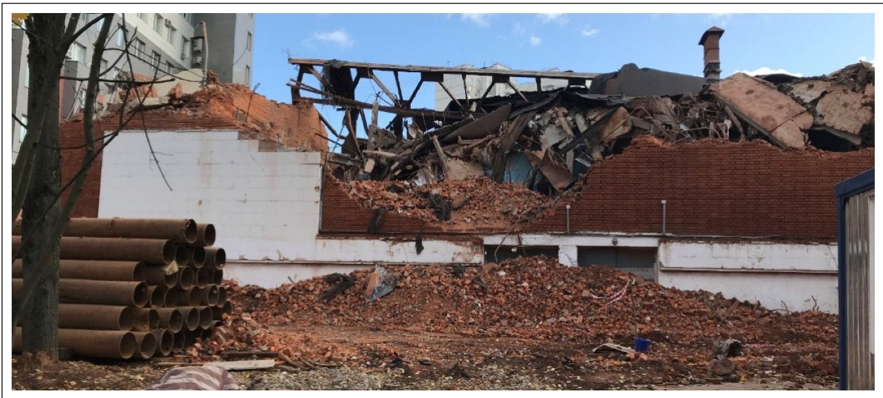
Figure 7. Steel roof trusses of the Vityaz Movie Theatre, captured during demolition.
