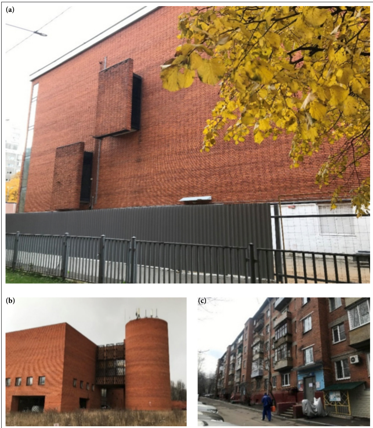
Figure 4. (a) The rear façade of the Vityaz Movie Theatre was captured during demolition. (b) Typical fenestration openings in brick façades across the city: Orlov Paleontological Museum (1965–1989), Moscow. (c) Five-story mass housing was constructed in Moscow in the 1960s and 1970s.
