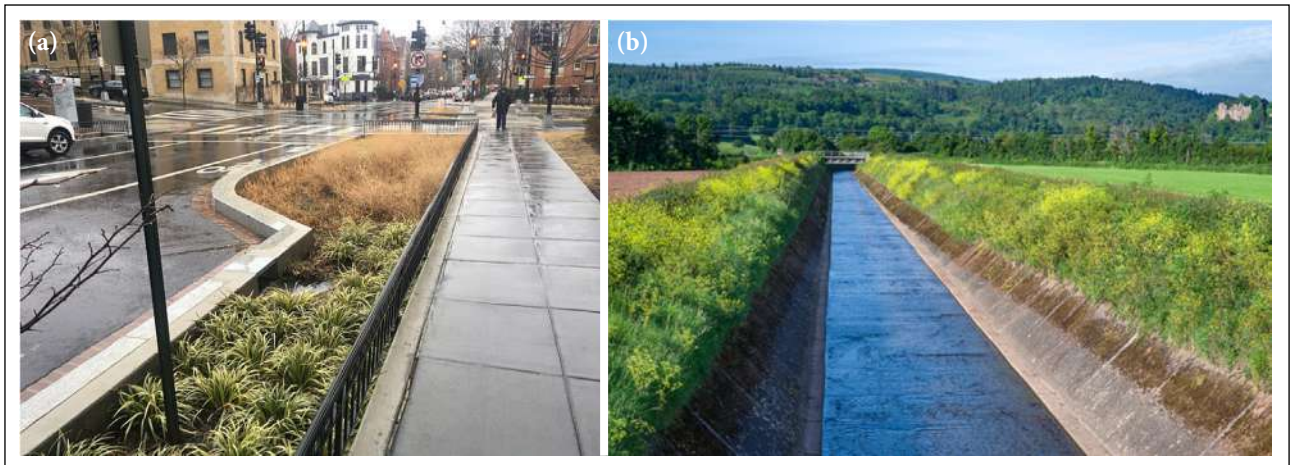
Figure 14. (a) Bioswale (left) and (b) Vegetated Concrete Channel (right).
